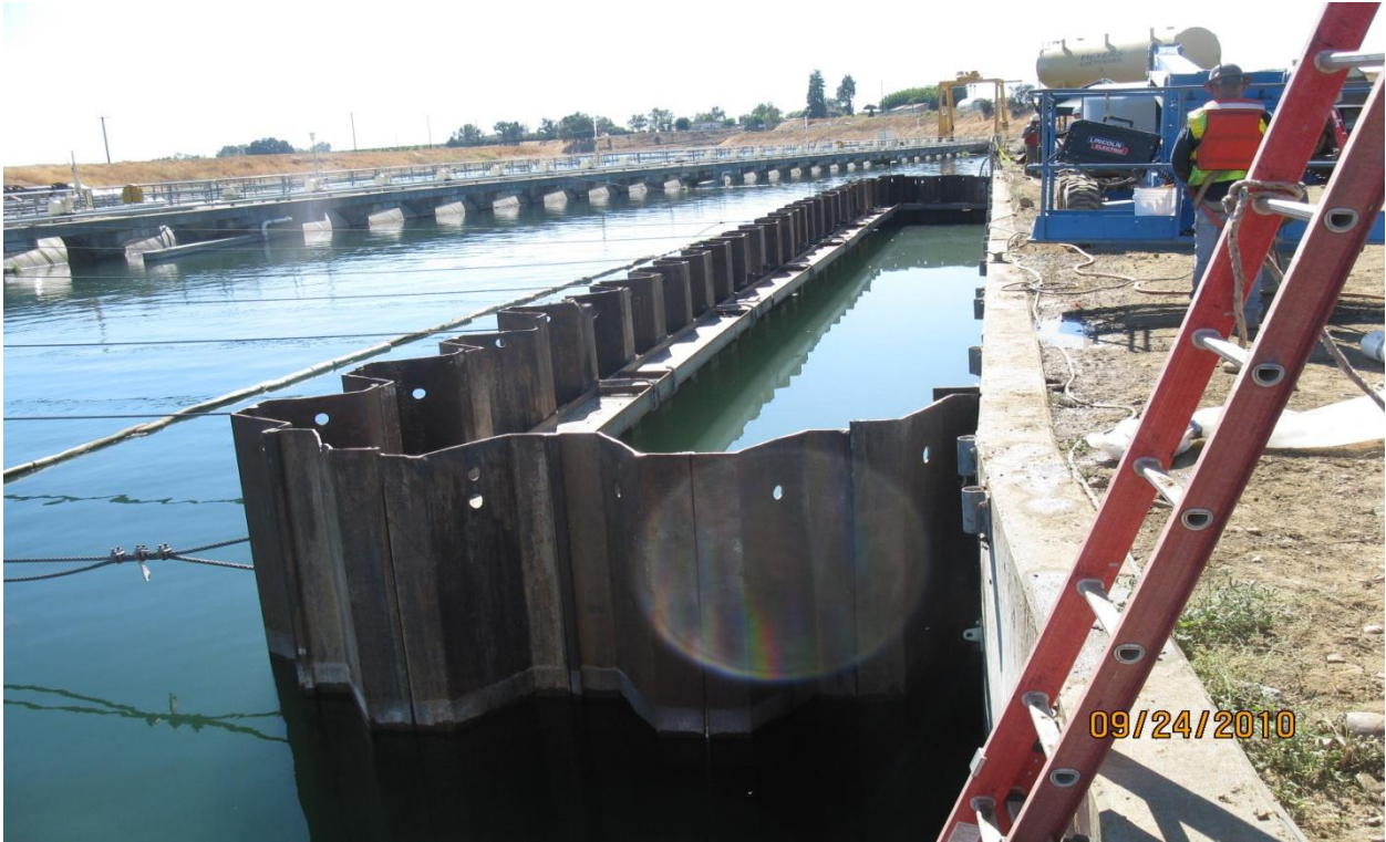
Coffer Dam for the Settling Basin Structure.
